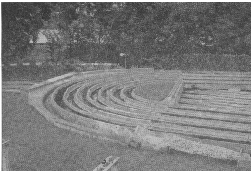
FIG. 6 ARTIFICIAL STREAM CONSTRUCTED OF CEMENT CANALS, ZURICH, SWITZERLAND
