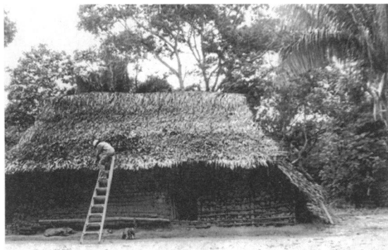
Fig. 1. Typical rural house used for the study showing the ladder employed to collect bugs on the roof.
