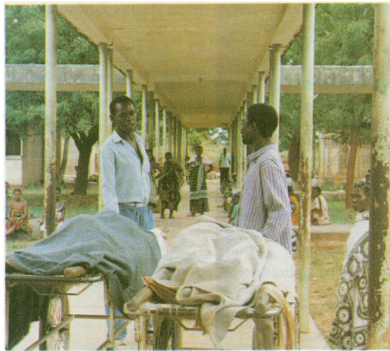
Concrete walkways connect the hospital's wards
