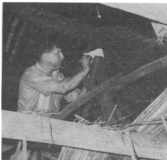
FIG. 2 FILTER-PAPER STRIP BEING PLACED ON VERTICAL ROOF BEAM
