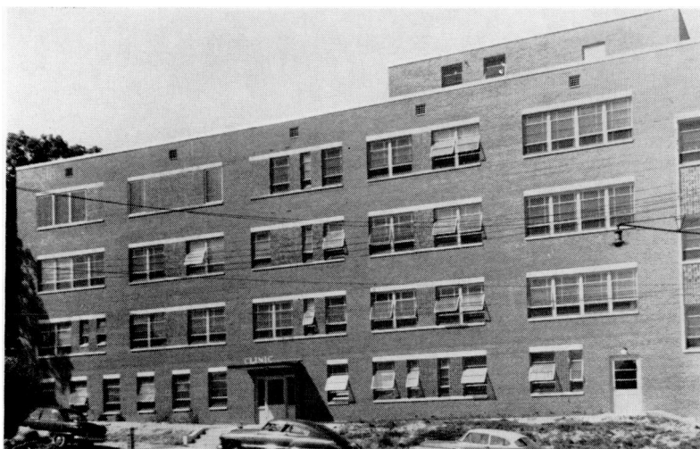
Side view of new $80,000 addition made possible through federal funds under Hill-Burton Act and additional funds authorized in Durham County Bond elections.
