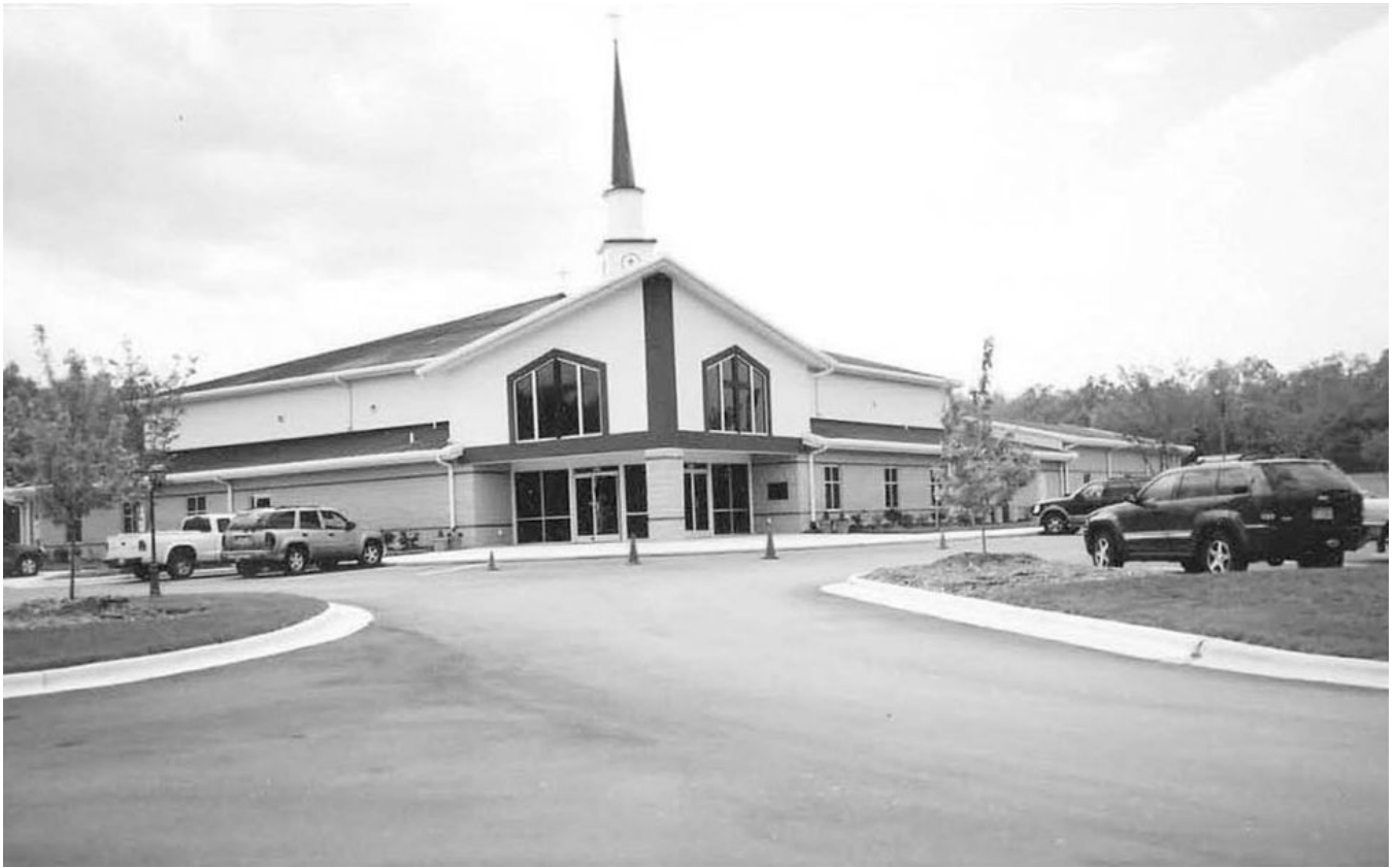
Figure 3. Photo of a Local Church
