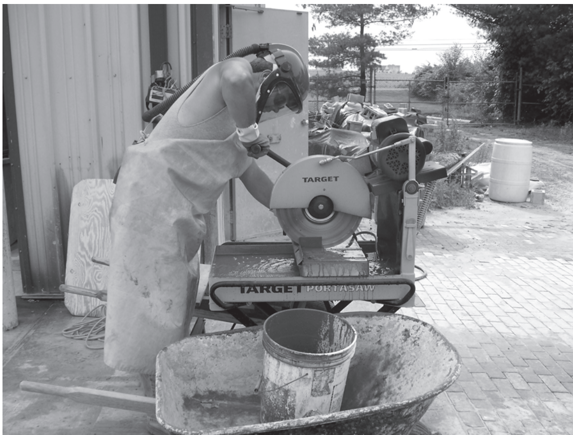
Photo 3. Brick cutting using Target® stationary wet saw
