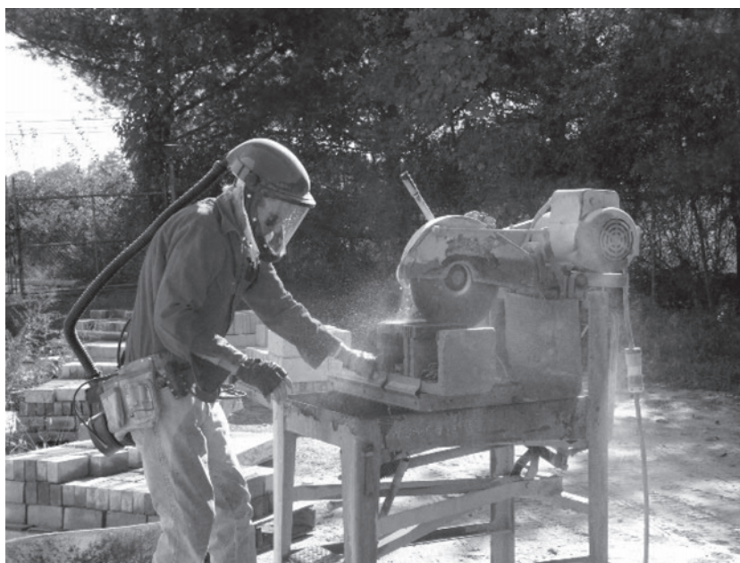
Photo 2. Block cutting using Felker ® stationary wet saw
