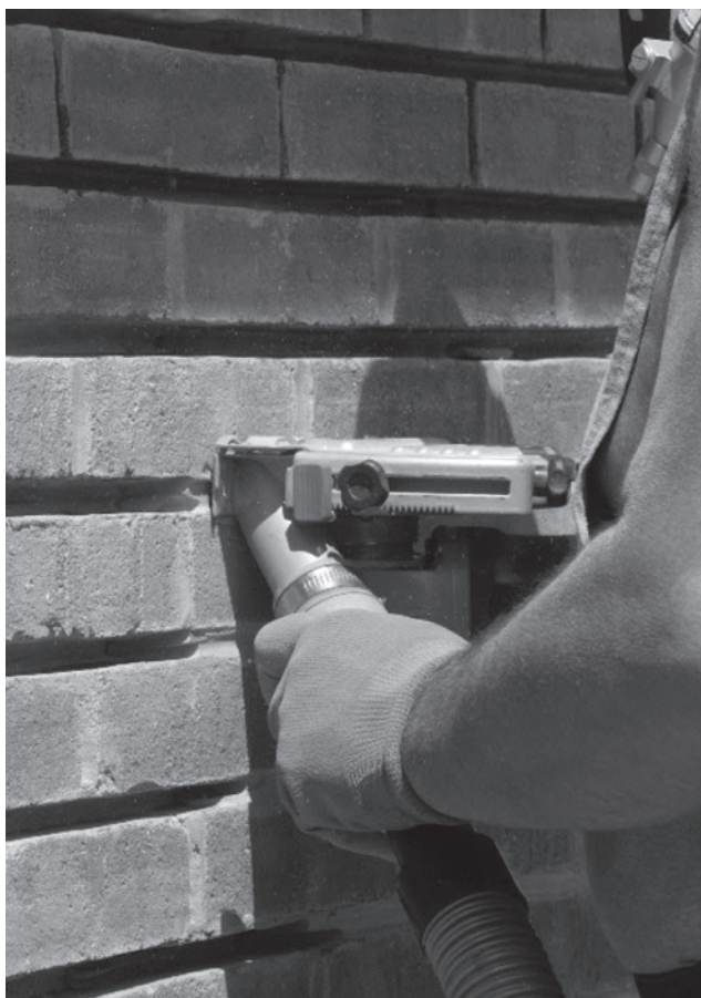
Photo 4. Tuckpointing using Bosch® grinder
