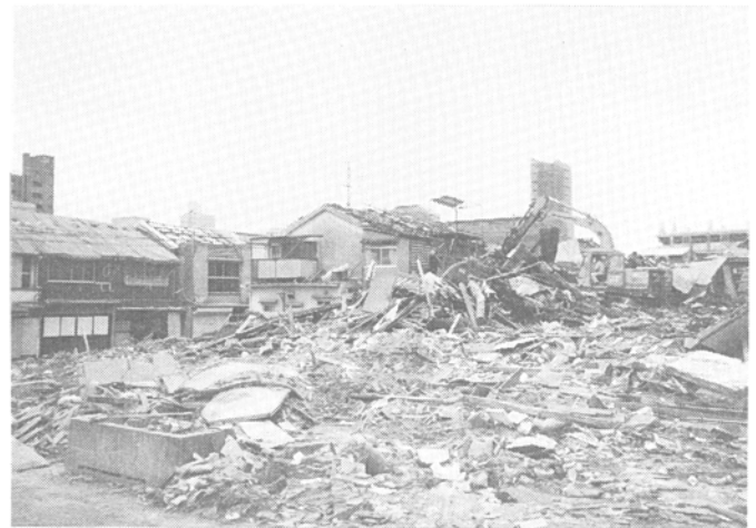
Fig. 3 Demolition of a wooden building.
