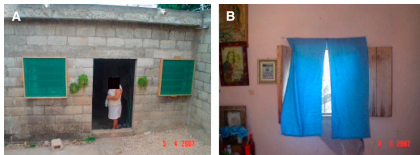
FIGURE 1. Examples of insect screens and impregnated curtains used. A , Insect screens were fixed on the outside of the houses. B , Long-lasting impregnated curtains were hung from a metal wire on the inside of the windows. This figure appears in color at www.ajtmh.org .
