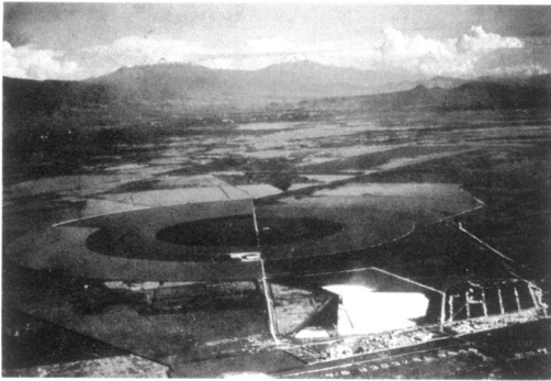
FIG. 5. Plant for the production of S. maxima on Lake Texcoco. S. maxima is harvested from the external portion of the 900-ha solar evaporator ( caracol ) built on Lake Texcoco, Mexico. (Photo courtesy of Sosa Texcoco S.A.)
