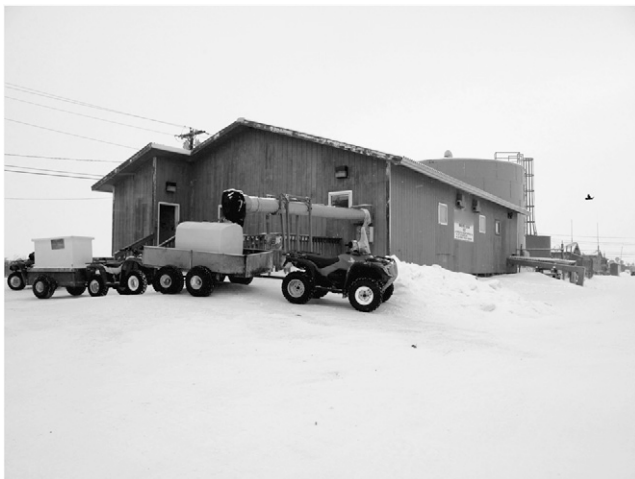
IMAGE 1—Four-wheelers from flush-haul households in line outside of Tundra Hill's washeteria, where residents use the large access point, protected by Arctic piping, to fill tanks or buckets with water to haul to their homes.
