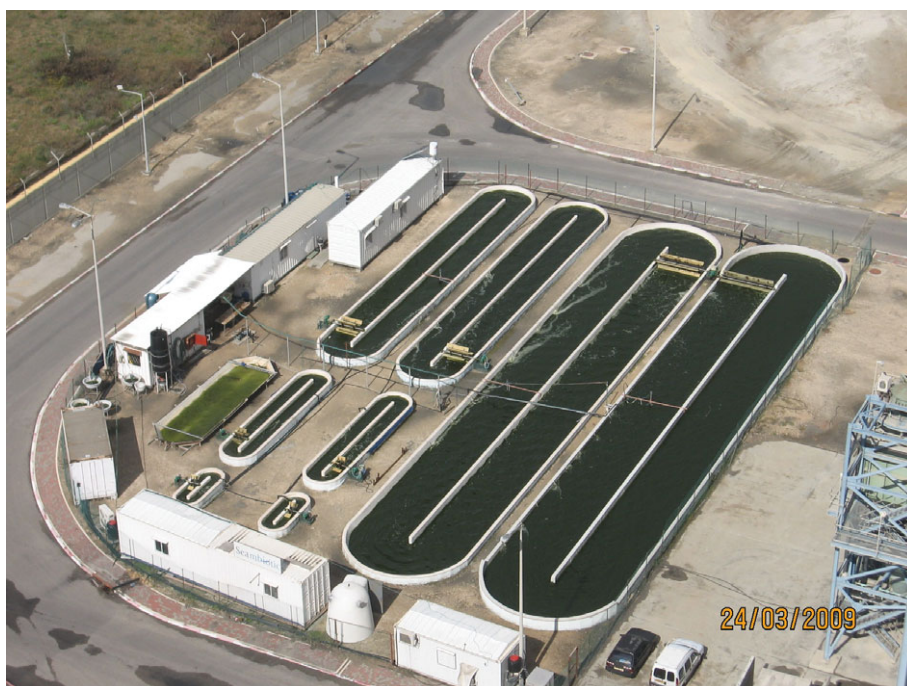
Figure 4. Image of large-scale Seambiotic Nannochloropsis sp. culture ponds. Image courtesy of Nature Beta Technologies Ltd, Eilat, Israel, subsidiary of Nikken Sohonsha Co., Gifu, Japan.
