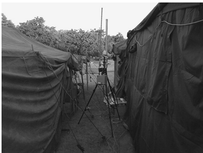
Figure 2 Wireless outdoor router used at the deployment.
