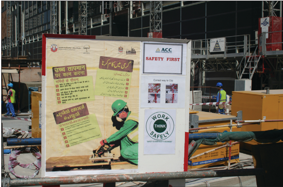
Example of Use of Awareness Posters in Multiple Languages at Construction Site in Abu Dhabi. Photograph by Darren Joubert.
