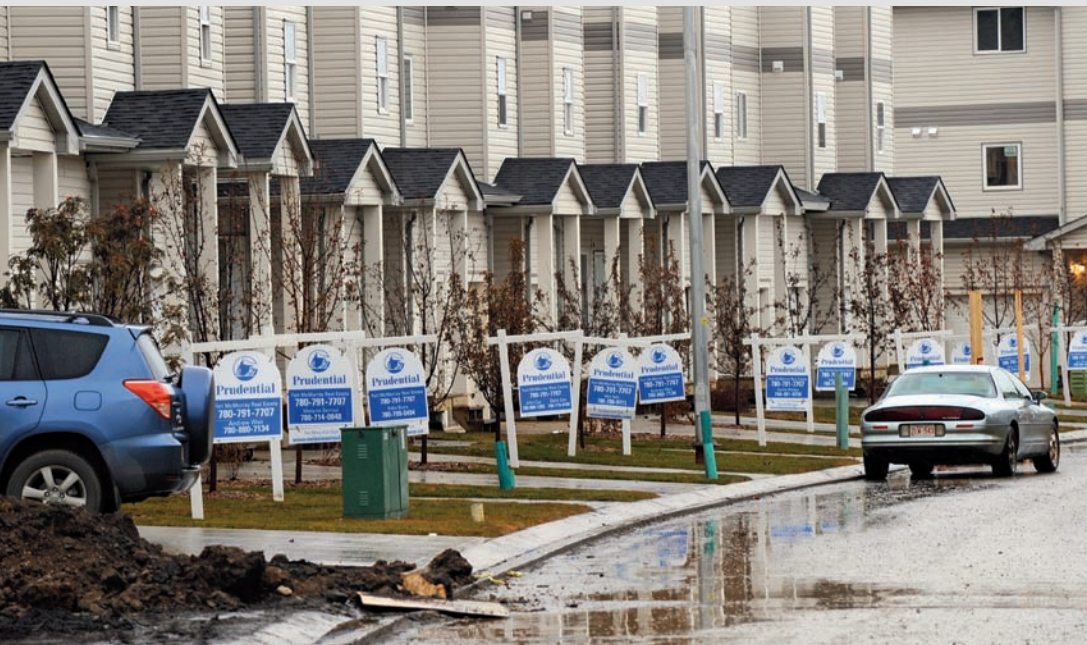
In late 2009 these houses were selling for around US$450,000 at a new property development in Fort McMurray, a boom town about 30 km south of the nearest oil sands operations. Transient workers with the oil sands and other industries make population estimates tricky, but by one estimate the population of Fort McMurray grew by 80% between 2000 and 2010, reaching nearly 77,000; it is expected to nearly double again by 2028. 26
