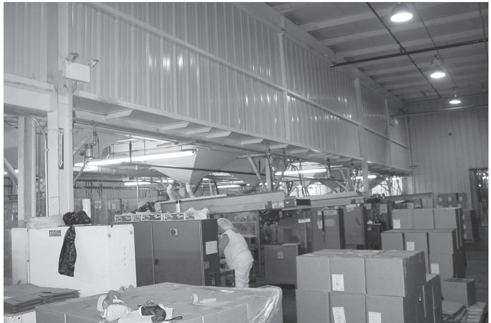
Photo 9: Mezzanine tank area walled off from the rest of the packaging line area. Courtesy of the National Institute for Occupational Safety and Health.
