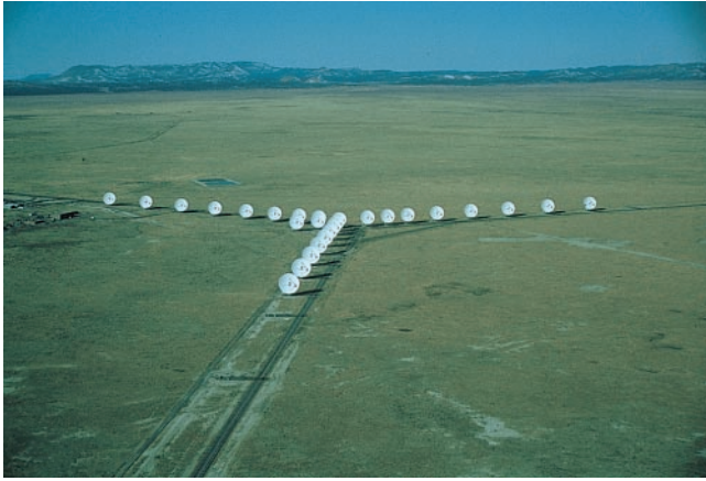
FIG. 2. The NRAO VLA is located on the Plains of San Agustin west of Socorro, NM. It has the angular resolution of a single filled aperture whose radius equals the length of each array arm, but its sensitivity is only that of 27 25-m telescopes. The individual telescopes can be moved to synthesize aperture diameters from 1 km to 36 km.
