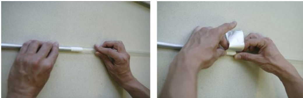
Figure 7. Attaching top extender - with PTFE (left) and reflective tape (right).
