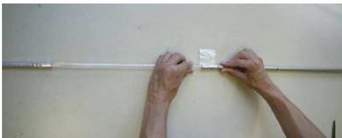
Figure 8. Attaching bottom extender - reflective tape.
