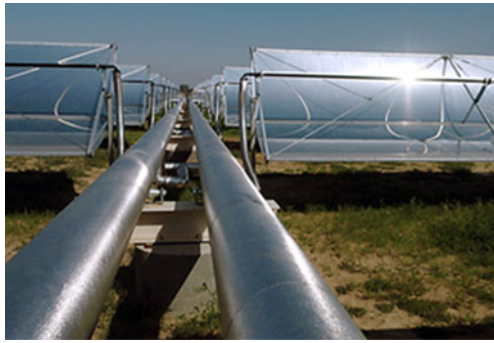
Fig. 5 Frito Lay “sun Chips” manufacturing unit at Modesto, CA (USA)
