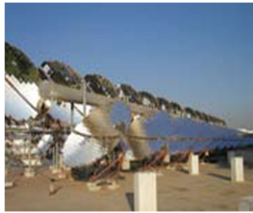
Fig. 4 An array of 84 Scheffler Reflectors of 10 m 2 each, Abu Road, Rajasthan for the kitchen at the centre of Brahma Kumaris
