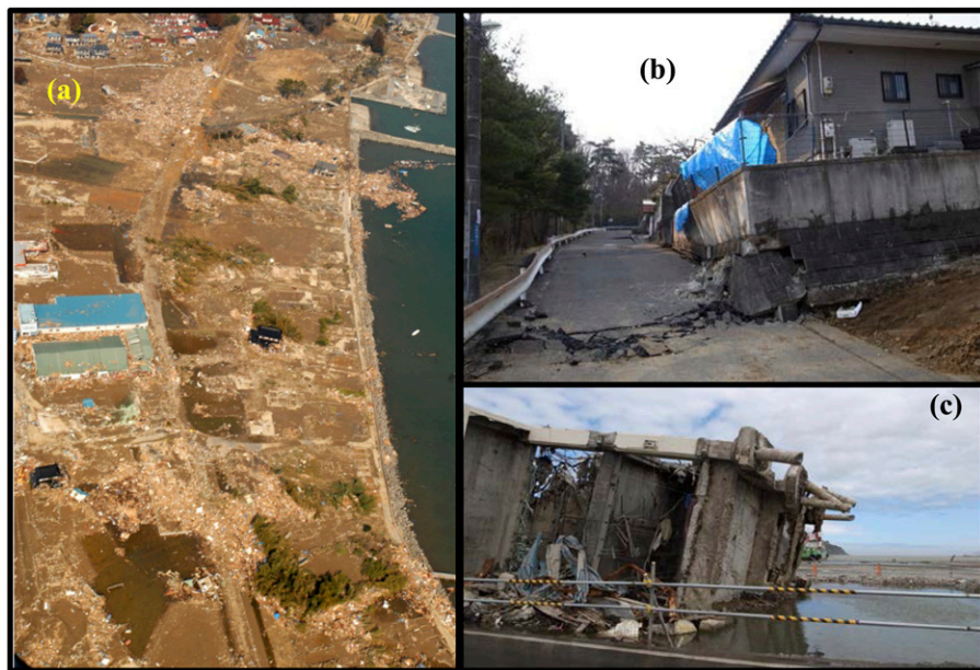
Fig. 5. Ecosystem impacts and urban/residential damage caused by the March 11, 2011, earthquake ( M = 9.0 ) and tsunami off the east coast of Japan. (A) Tsunami damage and potential ecosystem changes along the coastline north of Sendai (US Navy photo; D. McCord). (B) Homes and roads built on valley fills in Sendai destroyed by slope collapse (valley fill-type landslide). (C) Overturned reinforced concrete building with a pile foundation in Tohoku Prefecture, an example of a complex disaster where earthquake shaking liquefied the foundation ground and subsequent tsunami waves overcame resistance to pull-out forces.
