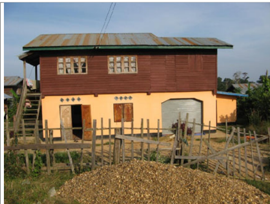
An improved house in Khammouane Province, south-central Lao PDR. The residents of the house have enclosed the open space below the house with brick and replaced wooden-shutter windows with glass. The walls and floors are constructed from pre-dried hardwood.
