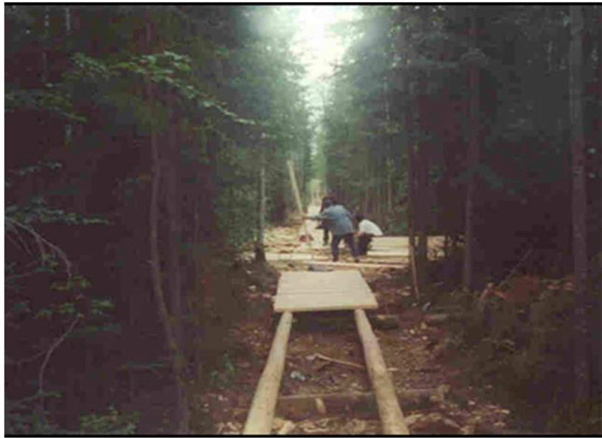
FIGURE 2 | Image showing a boardwalk portion of the walking trail under construction.
