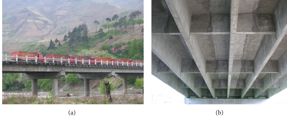
FIGURE 3: Overview of Nanping Bridge.
