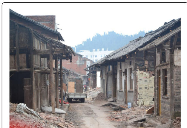
Figure 1 Collapsed houses in Guangyuan after the earthquake.
