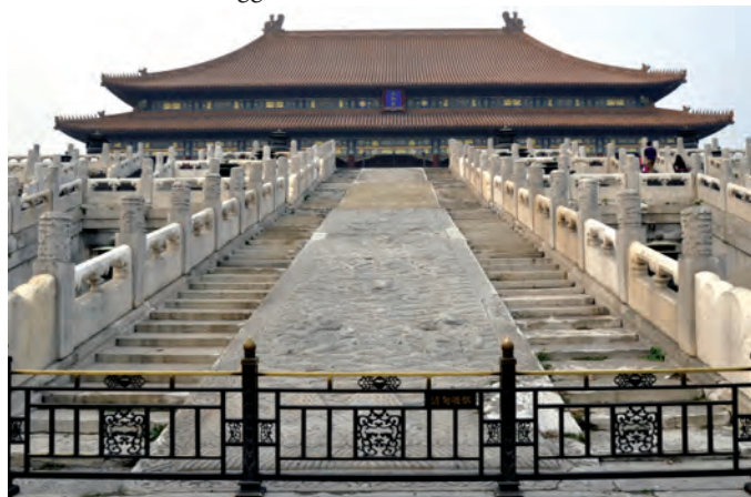
Workers likely slid massive stones, such as this 300-ton marble carving in front of the Hall of Supreme Harmony in the Forbidden City, Beijing, China, along artificial ice paths.
