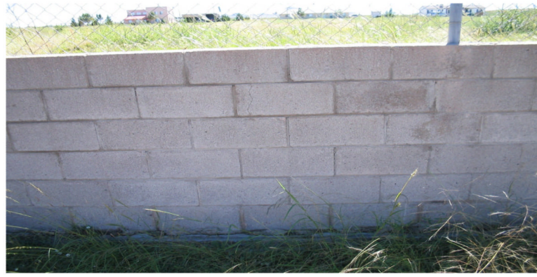
Figure 1. The Cinderblock Wall
