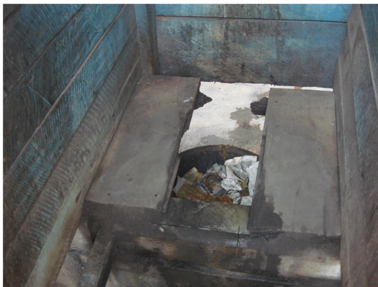
Figure 3 A bucket latrine: banned but still in existence. The latrine is a public toilet in one of the neighbourhoods.
