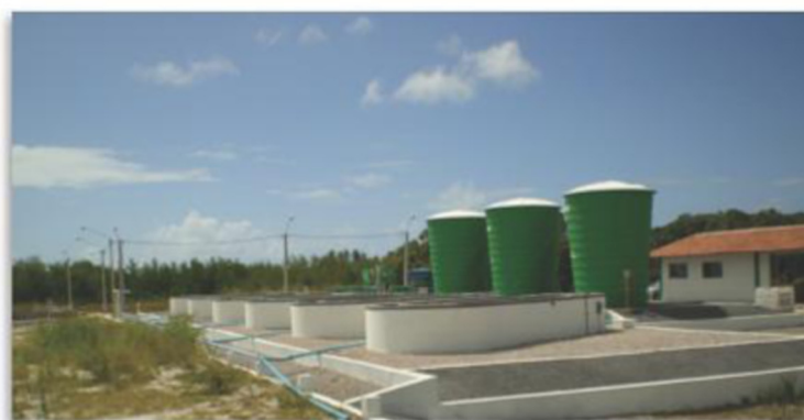
Figure 5 Microalgae pilot plant. A. Schematic diagram of the microalgae pilot plant for the production of biodiesel. At present the plant has the capacity to operate open ponds with a unit volume of 6,000 liters B. Photograph of the microalgae pilot plant for the production of biodiesel located in Extremoz at the Aquaculture Technology Center of UFRN (Universidade Federal do Rio Grande do Norte). Author's personal file, 2013.
