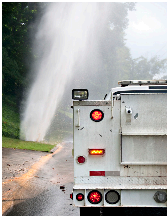
Pipe breaks and loss of water pressure provide opportunities for treated drinking water to become contaminated en route to consumers. © Eneri LLC/Gettyimages
