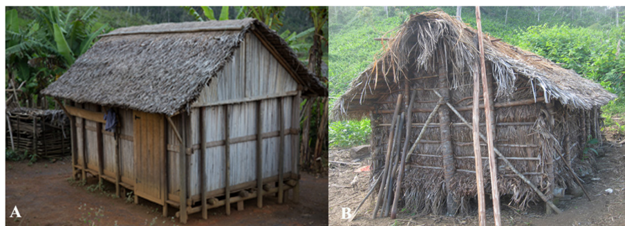
Figure 6 Housing structures built with R. madagascariensis . (A) Traditional house structure seen in Ambalabe using petioles for wall. (B) Temporary house structure built in the crop field with leaves used for roofs and wall.
