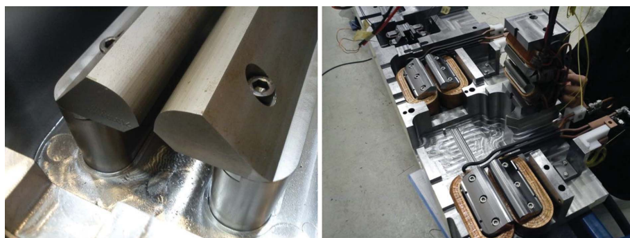
Figure 8 Left: M1 yoke bottom with QDend pole tips mounted on pole roots. Right: U4 magnet block top half being assembled. An SFo sextupole half is about to be installed between the two QF quadrupoles.
