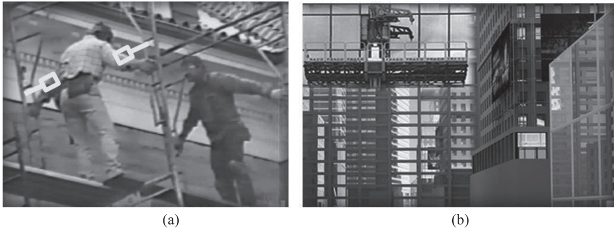
Fig. 6. (a) Scaffold-end-frame dismantling tasks require both muscle strength and postural balance skills (left). A set of tools or scaffold components (white bars) that encourages a hand separation distance of 46 cm would support workers to generate sufficient isometric strength to disassemble typical 23 kg scaffolds while concurrently allowing them to mitigate the likelihood of postural imbalance. (b) Mast climbing work platforms are increasingly being used in major construction projects in the U.S.
