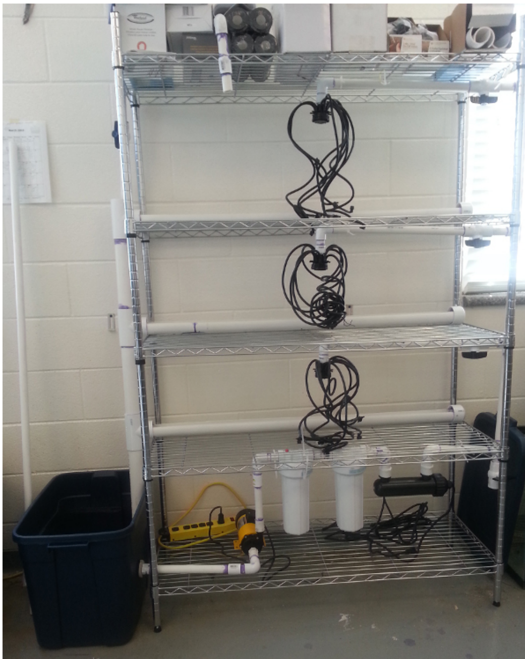
Figure 5: Completed system. The completed system contains a pump and filters system, a main vertical supply line, a horizontal supply line for each shelf, a tank exhaust line, a pressure relief line, and a main exhaust line for a contained circulation system.
