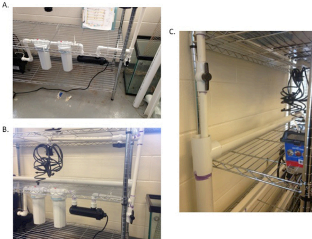
Figure 4: Individual parts construction. A. The three filter and pump system is on the bottom rack of the system. The pump is connected to three mechanical filters followed by a UV filter to eliminate contaminants from the system water. B. The horizontal supply line ends in a 9 port irrigation manifold, which will supply fresh water and oxygen to each tank. The supply line to each shelf has an on-off valve that can be used to stop water to each shelf for cleaning and quarantine purposes. C. The fish tank exhaust line empties into the main exhaust line to reenter circulation. The pressure relief line also empties into the main exhaust line.
