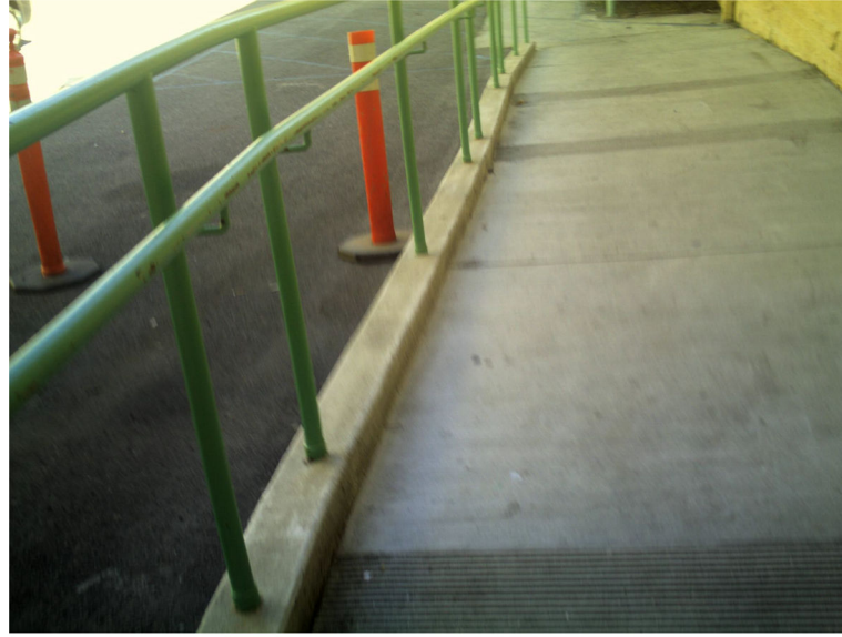
Fig. 3. Picture of ramp and handrails
