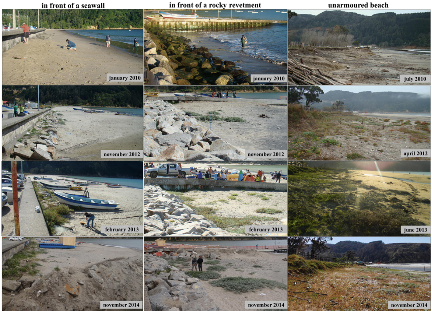
Fig 2. Before/after Maule earthquake (27th February 2010). Pictures of the armoured sites located in front of a seawall and a rocky revetment, and those of the unarmoured site taken at the beach of Lllico at different stages of the study. Note the increasing human activities at the seawall site and the developed vegetation at the unarmoured site after the earthquake. Repair work on the concrete wall affected the vegetated zone at that site during November 2014.
