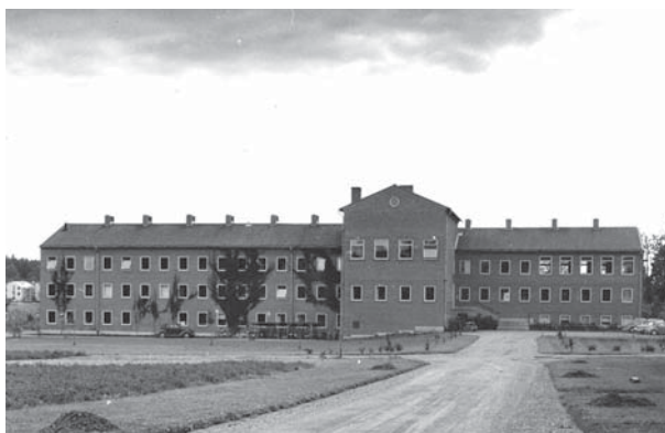
Figure 4. The Departments of Medical Chemistry and Pharmacology, located at Stockholmsvägen 19 (later named Dag Hammarskjölds väg).
