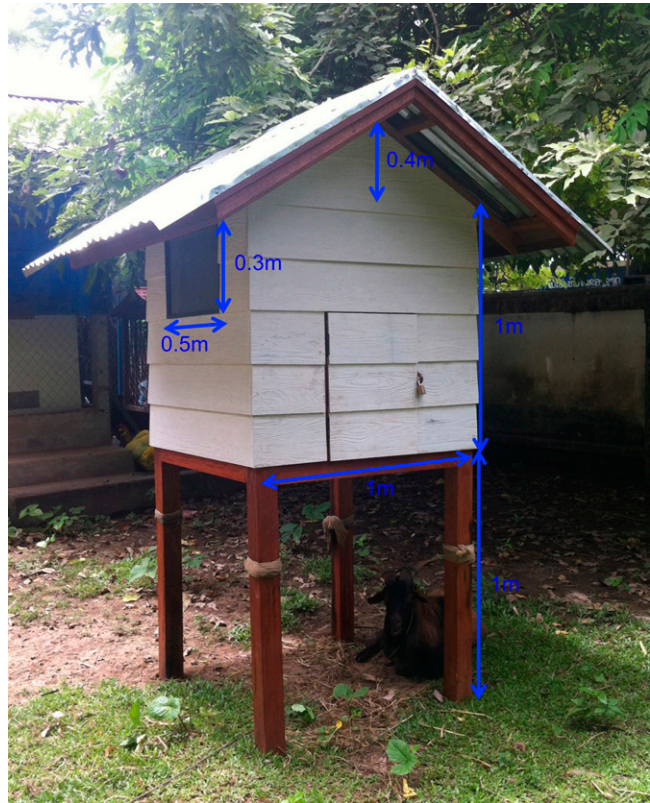
FIGURE 1. Hut for rapid diagnostic test (RDT) storage under field conditions. Hut constructed in wood to resemble miniature traditional Lao house. There is a goat beneath.
