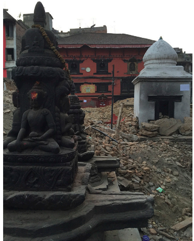
Collapsed temples in Bhaktapur Durbar Square in Kathmandu, Nepal. Photo by Michel D. Landry. Printed with permission.
