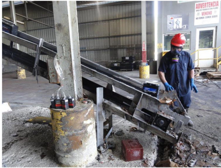
Figure 1. Area air sampling location 1 – sampling pumps were located by the battery breaker conveyor
