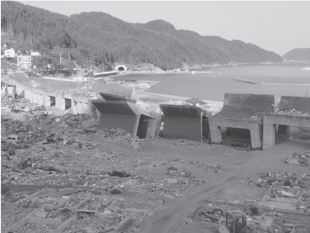
Fig. 3. Collapsed seawalls at Kojira-hama, Touni, Iwate Prefecture (June 19, 2011).
