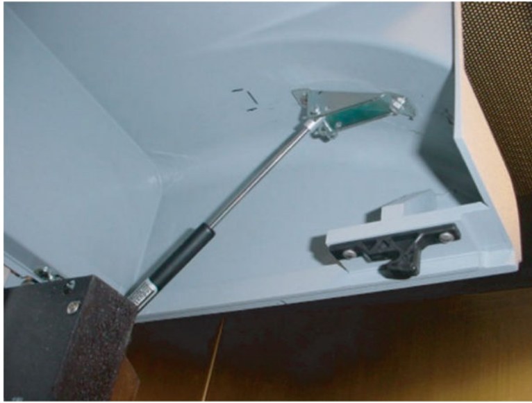
Fig. 1. Installation of a gas spring on the access door will permit the door to be easily opened and closed through the hood sash opening.
