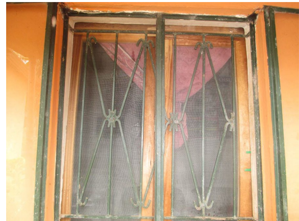
Fig. 2 A window with screening on one of the demonstration houses
