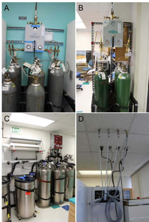
Figure 4. Sources of Gases and Power. (A) The CO 2 manifold is a 4 x 4 setup as it supplies all the incubators of the laboratory. (B) The O 2 manifold is a 2 x 2 setup and supplies only the cell production facility. Nitrogen for the system is generated in a vaporizer (C, just below the Exit sign) attached to a liquid nitrogen manifold (to the right) that also automatically fills cryofreezers (bottom left). The manifold is a 2 x 2 setup being supplied by two pairs of 160 L liquid nitrogen tanks. CO 2 , O 2 , and N 2 are supplied from the ceiling through shutoffs (D). House vacuum is also supplied at this location. Seen just behind the supply gas shutoffs are a pair of power cables that supply power to the system. Please click here to view a larger version of this figure.
