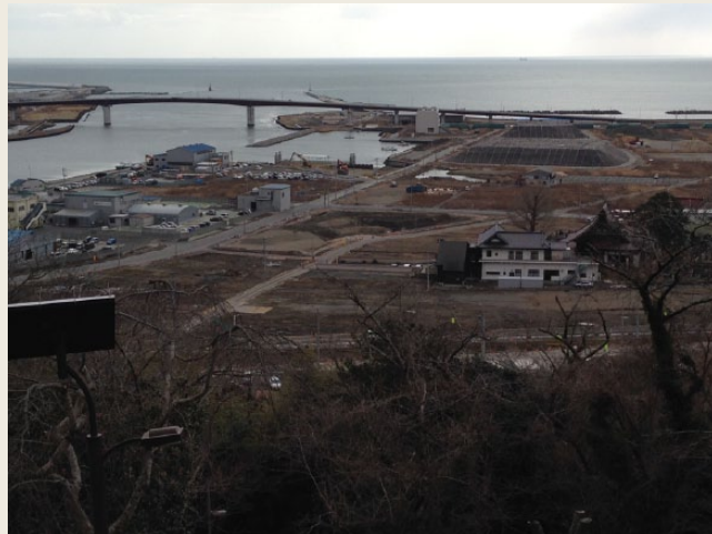
PHOTO 3 Comparing this picture to Photo 1 shows why this area of Ishinomaki is now called Bay of Destruction
