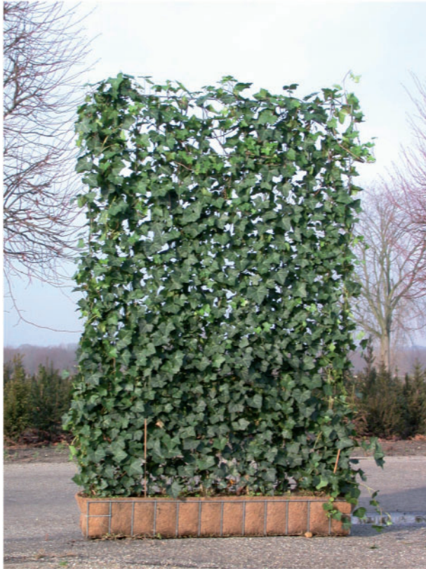
FIG. 8. Some green façades are designed to be mobile and used as temporary walls to create wind, solar irradiance and sound baffles. Photo courtesy of Sean Farrell, University of Staffordshire, UK.
