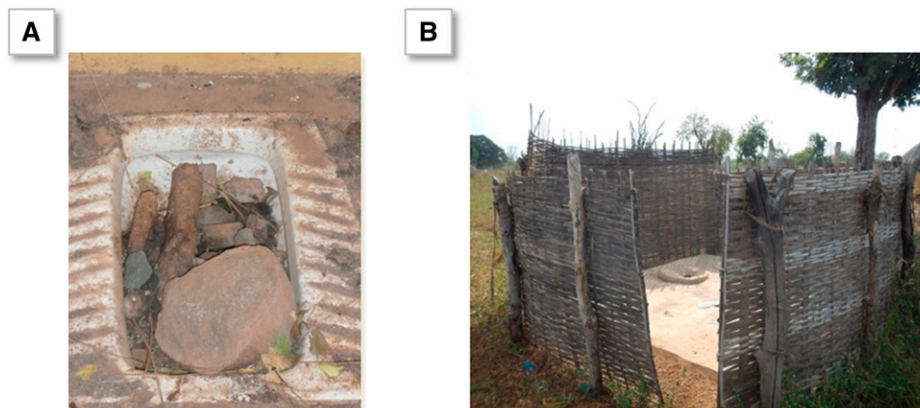
FIGURE 5. Latrine model and building. (A) Standard eastern-Senegalese-school-latrine model rejected by school-aged children was made with concrete blocks with a corrugated iron roof and inadequate waste pipes. (B) Latrine model accepted by inhabitants was made of a pit covered with a reinforced concrete slab, which was poured by a bricklayer. A fence around the latrine makes it possible to use it day and night.
