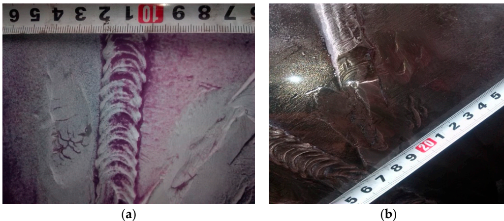
Figure 6. Inspections for external defects of pipeline girth weld: (a) dye penetrant; (b) magnetic particle.
