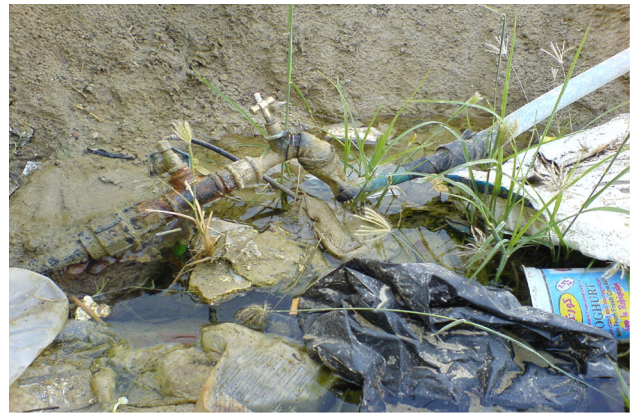
Fig. 3 Larval habitat due to damage and leakage of piped water network, southeastern Iran
