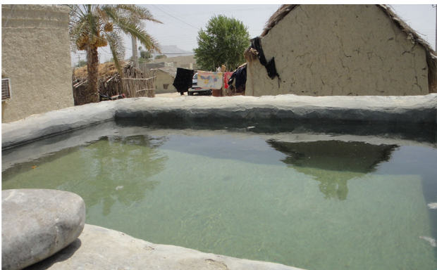
Fig. 2 The cement tanks (ponds) for using drinking and washing water before implementation of piped water network, southeastern Iran
