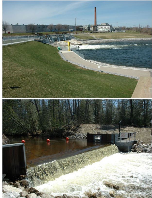
Figure 7: Sea lamprey barriers reduce the length of streams that need lampricide treatment. Hundreds of sea lamprey barriers are dams built for other purposes (hydropower, flood control, etc.) that fortuitously block adult sea lamprey spawning migrations (top). Additionally, barriers have been purposely built or modified to block adult sea lamprey migrations (bottom). Photo credits: M. Siefkes, Great Lakes Fishery Commission.
