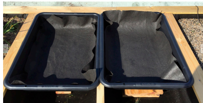
(a) Drainage Layer in the Green Roof Microcosms
